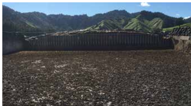
The silage pit showing the steel gates.
