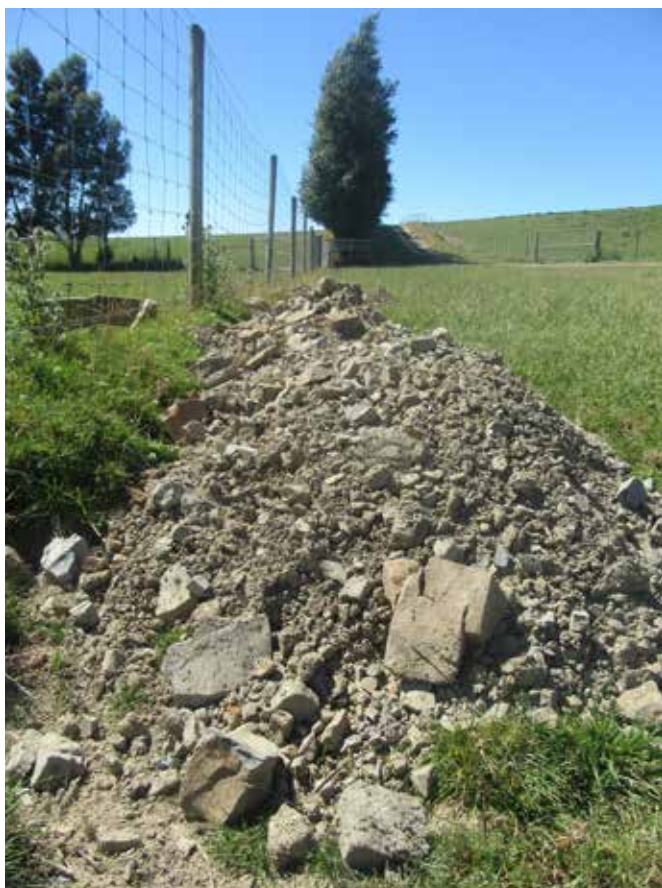
This rock buffer repairs the damage from fence pacing and helps prevent further sediment loss. Photo: Tim Fulton
