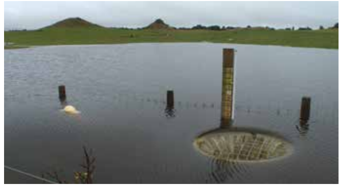
A detention bund at full capacity and skimming off excess storm water. Photo: Dylan Clarke.
