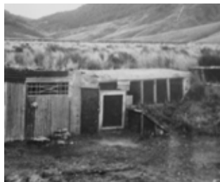
This meat safe constructed at Boyd airstrip by McNutt was used in the 1960s to hold deer carcasses before they were flown out.
