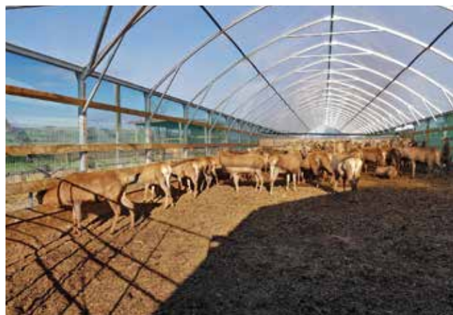
Bruce Allan’s Redpath shed: PVC roof allows the sun to warm up the interior.
