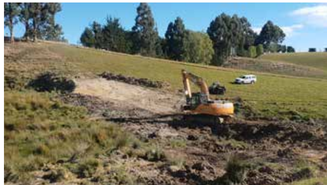
Earthworks establishing the restored wetland (above) and the developing wetland as seen by workshop visitors in August (below).
