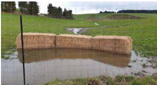
These straw bales make a good sediment filter. They can be secured in place with waratahs and are best kept out of reach of deer.
